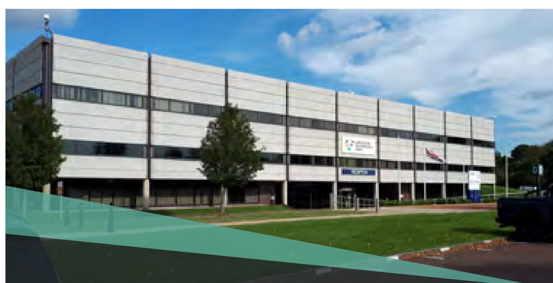
MANY BUILDINGS ON LANGSTONE PARK ARE UNSUITED TO MODERN BUSINESS NEEDS OR NEARING THE END OF THEIR SERVICEABLE LIVES
